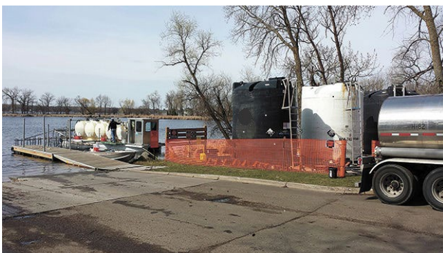
Figure 2. Staging Area and Tanks at Bald Eagle Lake, MN
